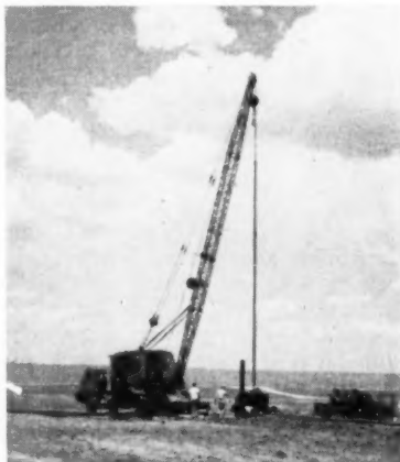
LOWERING casing down completed well. Wells average 460 feet deep.
